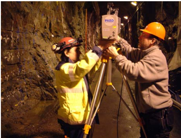
TASQ-tunnel, mounting of the Faro laser scanner used by ATS (photo Björn Magnor)
