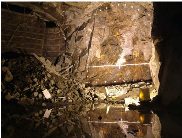
TASS-tunnel, geological mapping of the tunnel front, section 8.7 m (photo Carljohan Hardenby)
