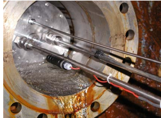
Installation of first model canister assembly
